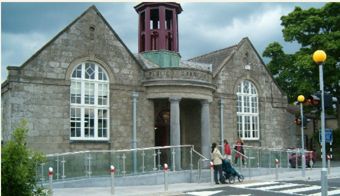
The new access ramp at the front door of Carnegie Library
